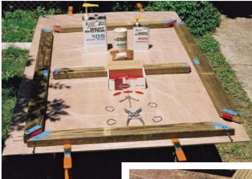
Figure 8. The gate's mitered corners are assembled with 4-inch stainless-steel screws, Lamello K-20 plastic biscuits, and two-part epoxy. Ulmia miter clamps from Garrett Wade (800/221-2942, [www.garrettwade.com](http://www.garrettwade.com)) hold the assembly together while the epoxy sets. The author prefers an intermediate rail to the more traditional diagonal brace because it matches the rest of the fence and provides space to mount the latch.
