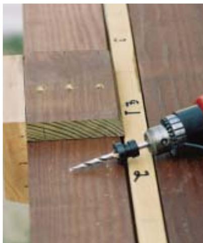
**Figure 5.** The screw pattern on the first full-sized fence board is laid out by hand, but then it becomes a jig for the rest of the boards when the author screws registration blocks on one end and one side (above). Smaller boards next to the post get their own jig. A WL Fuller Co. tapered bit (401/467-2900, [www.wlfuller.com](http://www.wlfuller.com)) does the drilling and counter-sinking in one step (left).
