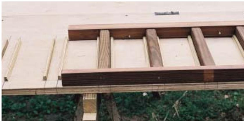
**Figure 4.** The 2x2 spindles capping the fence are laid into the jig and screwed to the rails with 3-inch-long #7 trim-head screws. The tops of panels are predrilled and screws are started to make final assembly easier (above). Keeping the spindles away from the posts helps hide slight discrepancies in the panel caused by warped posts and varying panel sizes (right).
