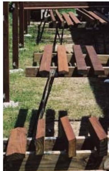
**Figure 2.** The top of every horizontal member gets a 15-degree bevel to shed water and debris. Rain grooves on the bottom of the top rail break surface tension so that water drips off instead of following the fence to the bottom.
