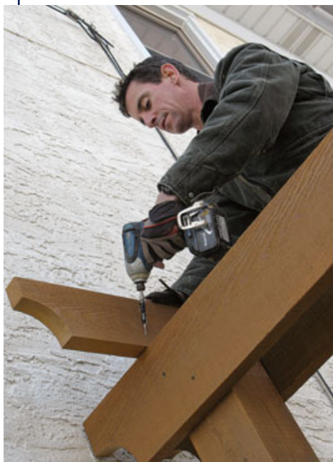
Figure 6. Rafter was toe-screwed to the girder with deck screws.
