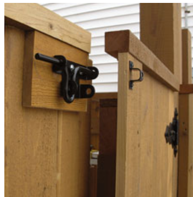
Figure 10. A standard gate latch holds the active side of the gate closed.
