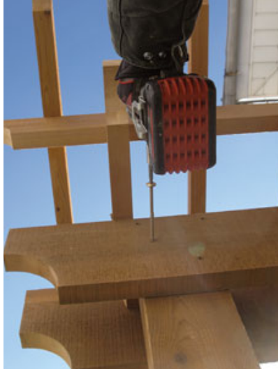
Figure 7. Six-inch-long “construction lags” fix the girders to the gate posts.
