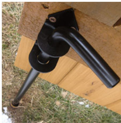
Figure 9. A cane bolt engages a pipe driven into the ground to secure the fixed half of the gate.
