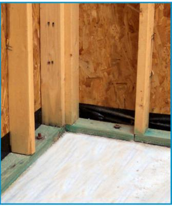
Advance Guard products are pressure treated with an EPA registered borate wood preservative, disodium octaborate tetrahydrate (DOT) for protection against termites, carpenter ants, fungal decay and dry rot.
