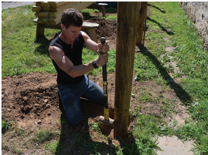
Figure 3. Compacting the soil while backfilling prevents settling around the post and provides it with extra support (top left). The 2x6 PT planks are fastened to the posts with 3-inch-long structural screws (center left). After setting his saw's cutting depth to the thickness of the planks and snapping a line, the author cut them to length in place (bottom left).
