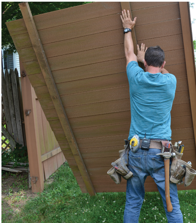
Figure 1. Installation started with demolition of the existing fence. After separating the panels from the posts, the author sawed the posts off just below grade, rather than try to remove them.
