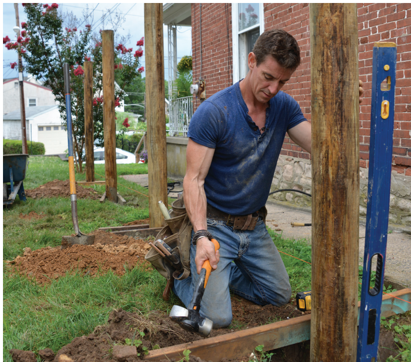
Figure 2. The author hammered pairs of 2x4 stretchers into the ground to temporarily hold the plumbed 6-inch-diameter PT posts in position while pouring concrete around the post bases. The post holes are 36 inches deep, or frost depth.
