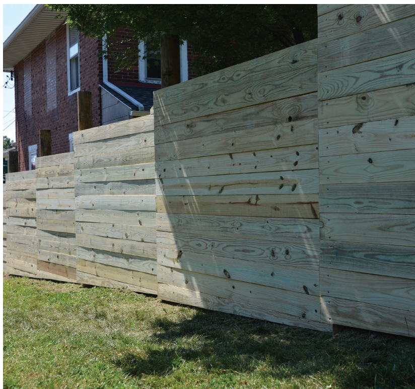
Figure 6. Because 2x6 PT lumber isn't perfectly flat, it creates interesting shadow lines in the fence. For a smoother surface, vertical cleats could be screwed to the backs of the panels to pull the boards into alignment.
