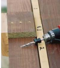
Figure 5. The screw pattern on the first full-sized fence board is laid out by hand, but then it becomes a jig for the rest of the boards when the author screws registration blocks on one end and one side (above). Smaller boards next to the post get their own jig. A WL Fuller Co. tapered bit (401/ 467-2900, www.wlfuller.com) does the drilling and countersinking in one step (left).
