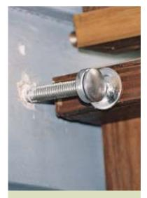
Figure 7. In the New Orleans area, wood structures cannot be attached directly to a house, so the author secures fence sections abutting the home with stainless-steel carriage bolts that pass through eyebolts into brass inserts epoxied into the framing. This method prevents direct woodto-wood contact and allows inspection during annual termite treatments.
