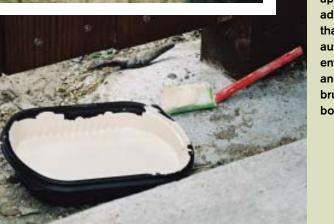
Figure 9. Designed primarily for industrial applications, two-part coatings have better adhesion and a higher percentage of solids than conventional one-part paints. The author uses them to prevent water from entering vulnerable end grain (above left and right). Bending the handle on a foam brush makes coating the bottom of fence boards easier (left).
